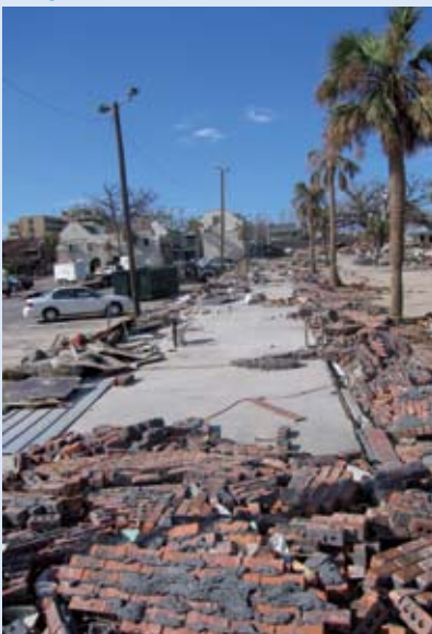
Damages from Hurricane Katrina, © Munich Re
